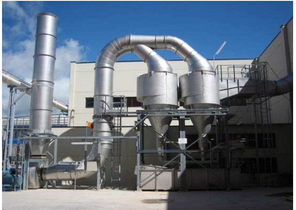
The exhaust gas extraction system is installed on the continuous press in charge of panel production in order to minimize the risks of fire.
